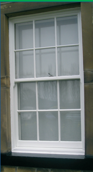
The repaired window is painted.
